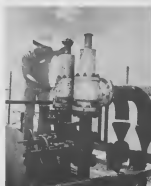
Clyde checking geeket leaks on pipelines in the Oil Movements eree.
